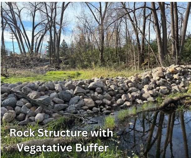
Stabilizing the ravine
